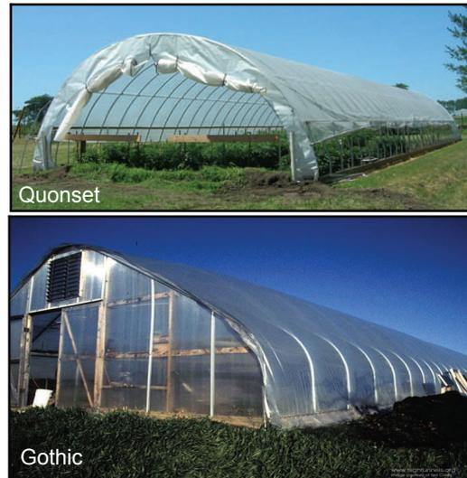
**Figure 2.** High tunnel shapes.
