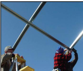
**Figure 4.** Purlins and the ridgepole connect the ribs together for support and strength.
