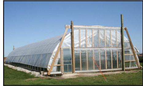
**Figure 1.** High tunnels are simple, plastic covered, passive-solar-heated structures.
