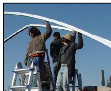
**Figure 5.** Several hands are needed to hold the metal bows or ribs while they are being installed.
