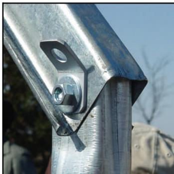
**Figure 3.** The metal bows are attached to the side posts.
